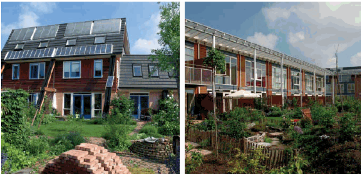
Fig. 50 Innovative housing: examples of private housing initiatives. Left: Semi detached houses with sun panels for photovoltaic and heating. Right: Row houses with joint landscaping. Source: VROM [77]
