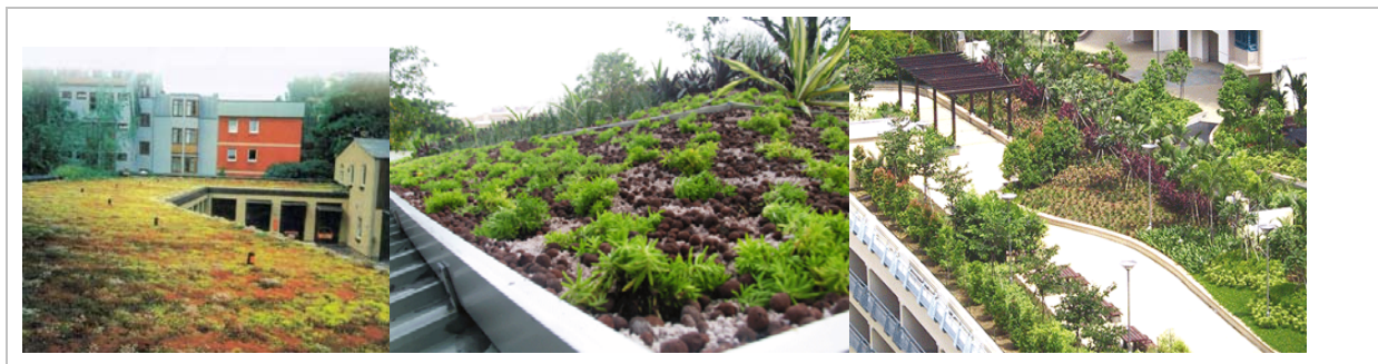
Fig. 76 Green roof types: extensive, semi-intensive, or intensive
