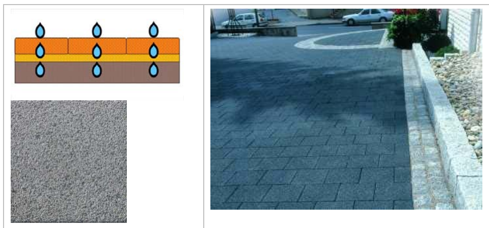
Fig. 73 Left: principle of permeable concrete blocks, right: parking area with permeable concrete blocks
